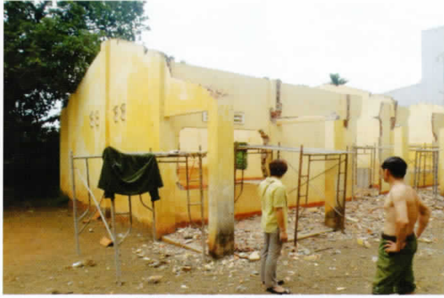
Building new dining room
